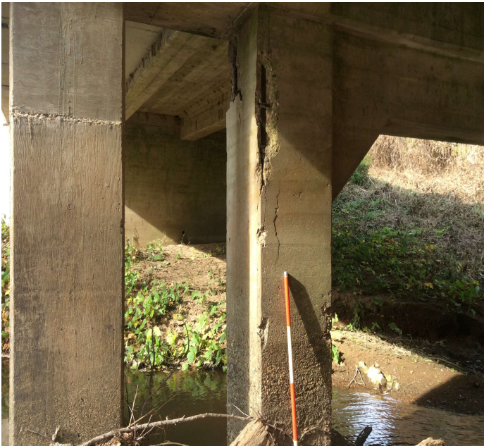
PHOTO 1 Description Bent 2 column 3 lager spall with exposed rebar
